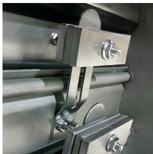
Counterbalance weights mounted to damper blades
