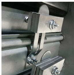
counterbalance weights mounted to blades
