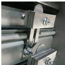
counterbalance weights mounted to blades
